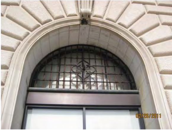
(f) Detail of ironwork at door
