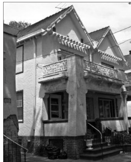
Tile roof restoration at 2418 S. 21st Street (Girard Estate).
