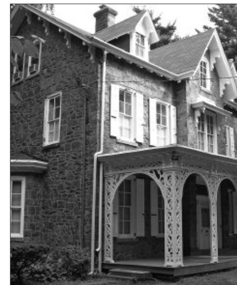
Restoration of porch, cornices, eaves and gutters at 639 Church Lane (Germantown).
