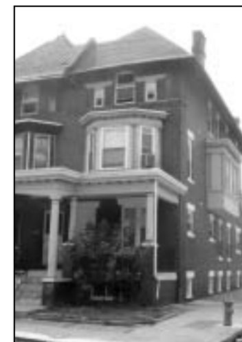
Partnership CDC rehabilitation project.
