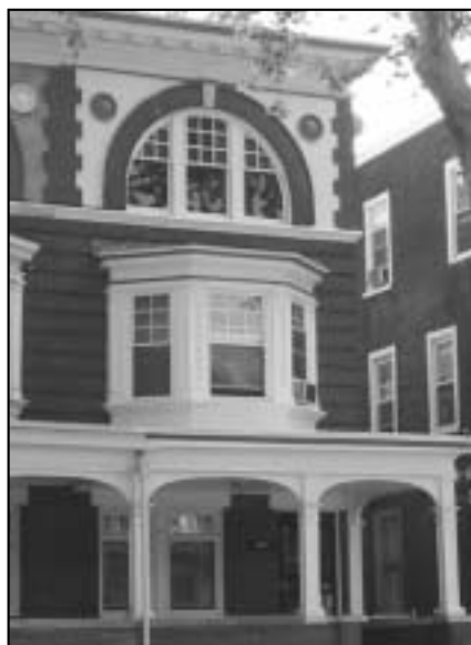
Partnership CDC rehabilitation project.
